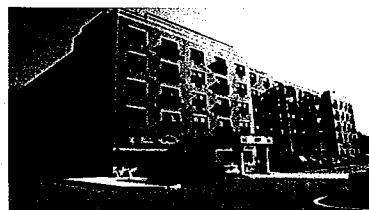
North Center Senior Housing, Chicago
